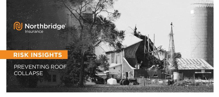
Extreme weather conditions, general wear and poor maintenance can jeopardize the structural integrity of industrial and commercial buildings. The accumulation of snow and ice places stress on all types of roofs. In farm buildings specifically, corrosive materials can build up to weaken the gusset plates that bind the trusses together.
